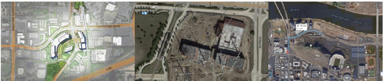
State Farm’s three new regional hubs. Atlanta (left) rendering courtesy of State Farm; Dallas and Tempe from Google Earth. Read more at http://t4america.org/2015/03/16/state-farm-is-moving-to-concentrate-thousands-of-employees-in-locations-near-transit/ .
