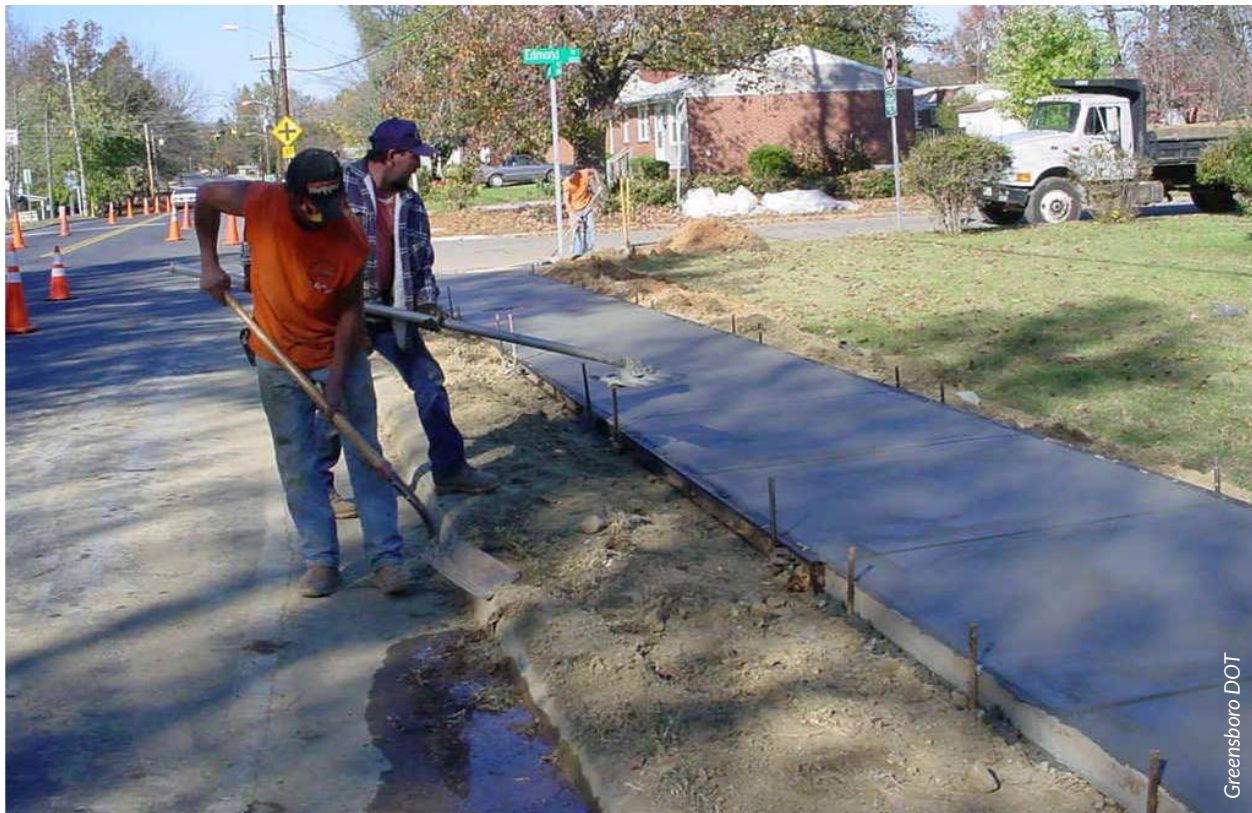
Workers construct a sidewalk on Willow Road.
