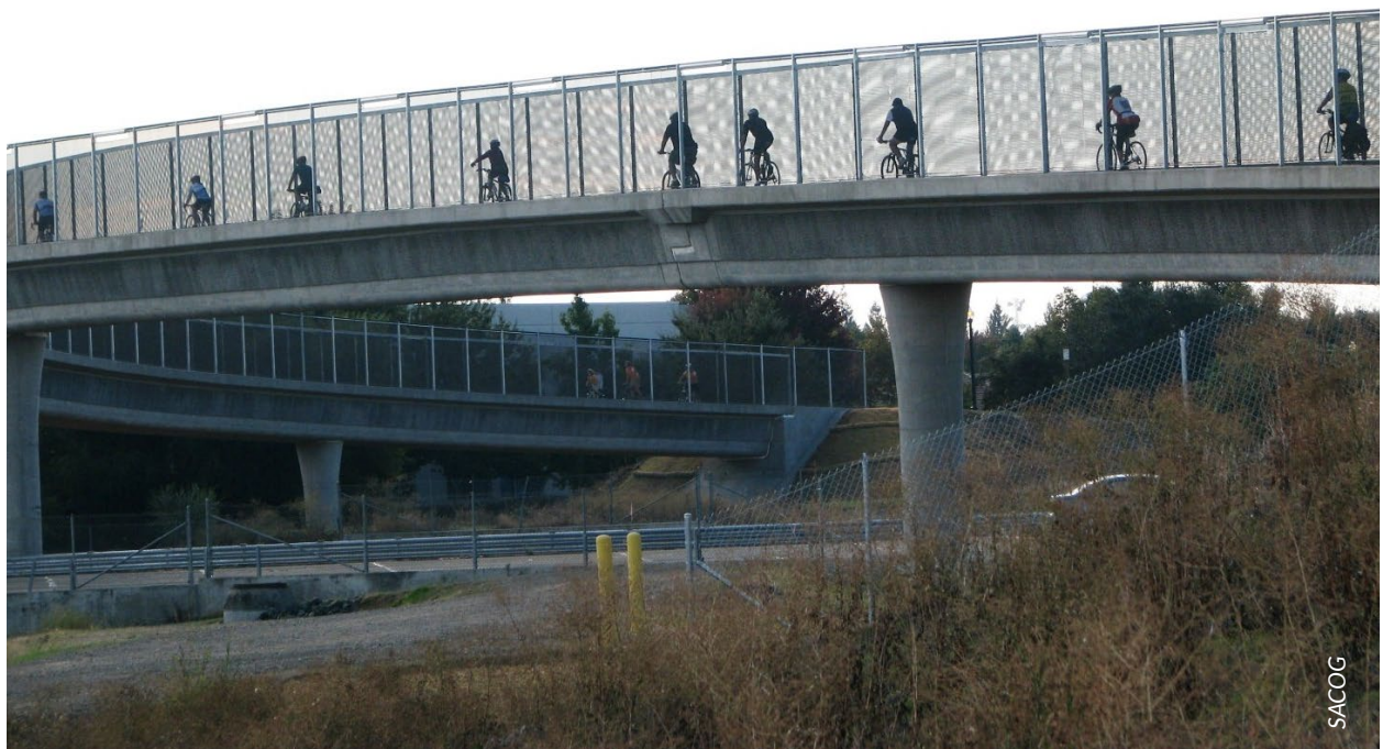
Bicyclists use an overpass across I-80 in Sacramento, a vital link that connects hundreds of miles of bike trails throughout the county and region.
